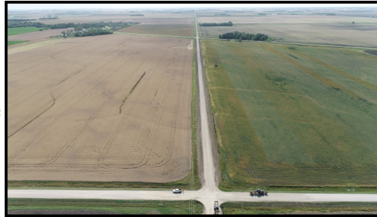
Gendron Road Rebuild (Between Diversion Rd & PR 210)
